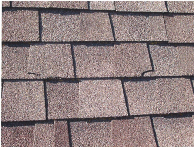
11. DAMAGED SHINGLES
