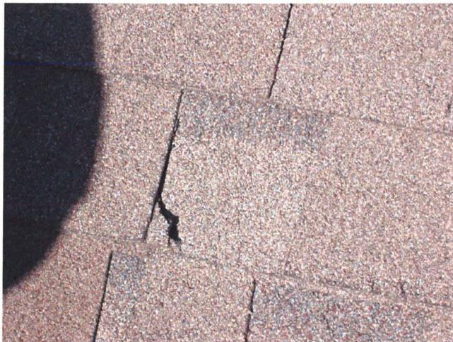
9. CRACKED SHINGLES
